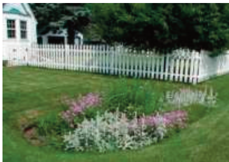
A rain garden with no berm
